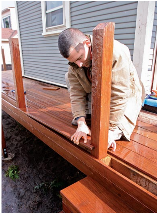
Streamline the post connection. The top riser is continuous with the deck's fascia for a clean transition. The outside course of decking is full width and is notched around each newel post.
