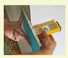
More accurate outside corners. A scrap of wood or drywall held flat against the wall makes an accurate outsidecorner measuring surface.
