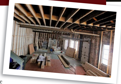
No load-bearing partitions here. Steel I-beams and sistered rafters reinforce the roof, leaving a wide-open floor plan. Placing the entry foyer where the loading dock was makes use of an existing opening. Maintaining the long view makes the narrow space feel much larger than it is. High-efficiency appliances, fluorescent fixtures, and ample daylighting help to keep utility bills low. FSC-certified flooring, trim, and framing lumber; bamboo plywood cabinets; recycled-content tile; and PaperStone counters add to the building's sustainable interior.
