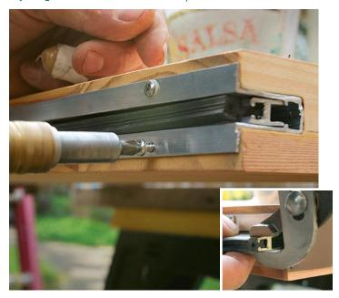
Secure with screws glued in place. After sealing the inside of the groove and the door bottom with polyurethane sealant, I position the mechanism, drill pilot holes, and attach it with screws. I squeeze a small amount of wood glue into each hole before securing each fastener. I secure the bumper by crimping the aluminum bar at one end.
