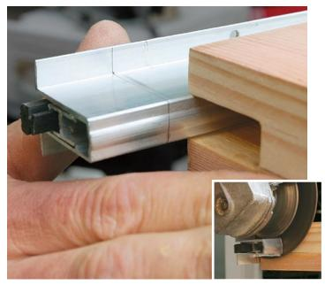
Cut the seal and housing in one step. After I've checked the mechanism's fit in the groove and scribed it to match the width of the door, I move the scribe line clear of the door's edge and cut the entire mechanism to length with an abrasive grinding blade (a fine-toothed hacksaw will work as well). Note: The neoprene bumper can move laterally inside the housing, so before you cut, make sure its opposite end is flush with the end of the housing.
