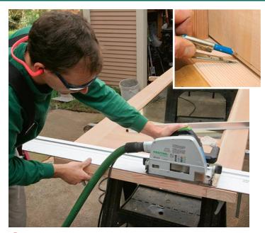
Trim the door bottom. For the weatherseal to operate correctly, the bottom of the door must be no more than ½ in. above the top of the threshold. After marking this dimension on both the hinge and latch sides of the door bottom (inset photo), I trim the door using a circular saw and a straightedge guide. For a review of different guides, check FHB #182, or online at FineHomebuilding.com.
