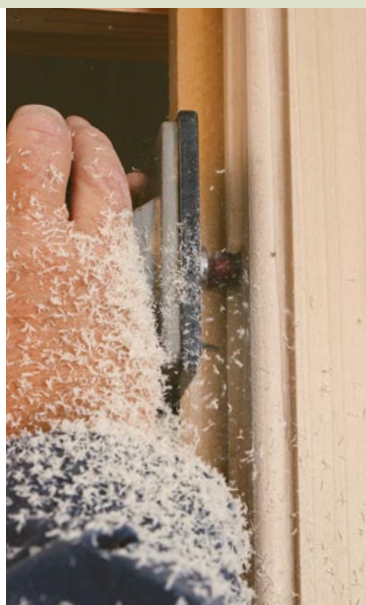
Plow a mortise
