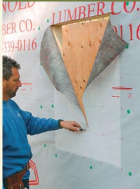
First, cut across the header, then down the center.
