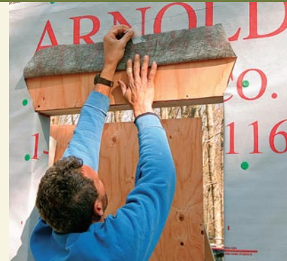
Fold up the top tab, and tape it out of the way.
