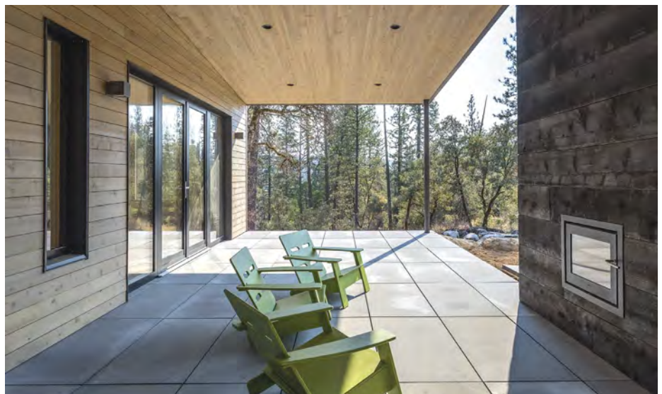
Sheltering room. StepStone concrete pavers at finish-floor height extend the indoors out, while the wall-like chimney and fireplace will ward off a chill.
