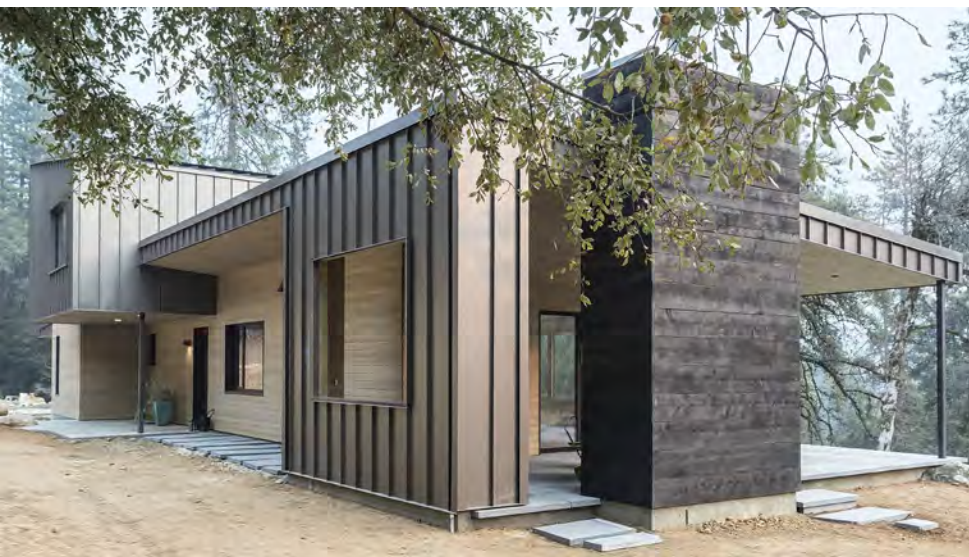
A charred chimney. The Shou Sugi Ban treatment of the cedar creates a cladding that is resistant to rot and decay and that highlights the grain pattern.
