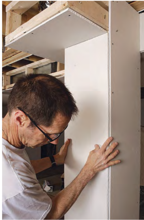
Mind the gap. Attach one piece of drywall flush with the corner, then attach the next piece up to 1/8 in. back from the corner so that the corner bead can sit flush on both sides.
