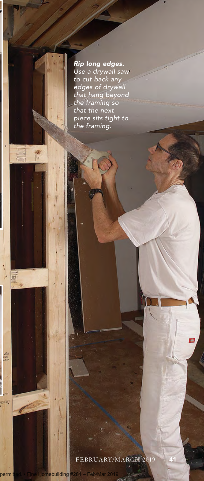
Mind the gap. Attach one piece of drywall flush with the corner, then attach the next piece up to 1/8 in. back from the corner so that the corner bead can sit flush on both sides.
