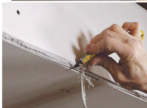
Bevel the edge. To cut back overhanging edges in places too tight for a drywall saw or where a drywall saw might damage the adjoining drywall surface, use a utility knife to create a chamfer.
