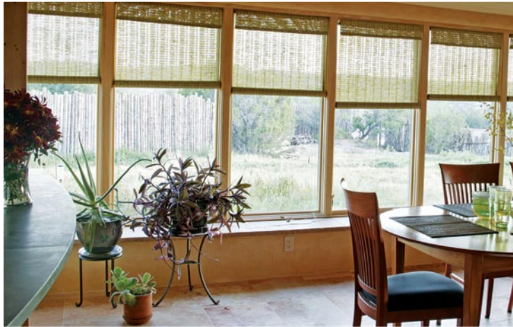
CATCHING—NOT DODGING—THE SUN Unlike the rest of the windows in the house, which are set back under a 4-foot overhang, the 24-foot bank of windows in the south-facing dining room come to within 18 inches of the edge of the roof to catch the sun's warming rays. The stone floor in front of the window absorbs heat and radiates it back into the house.
