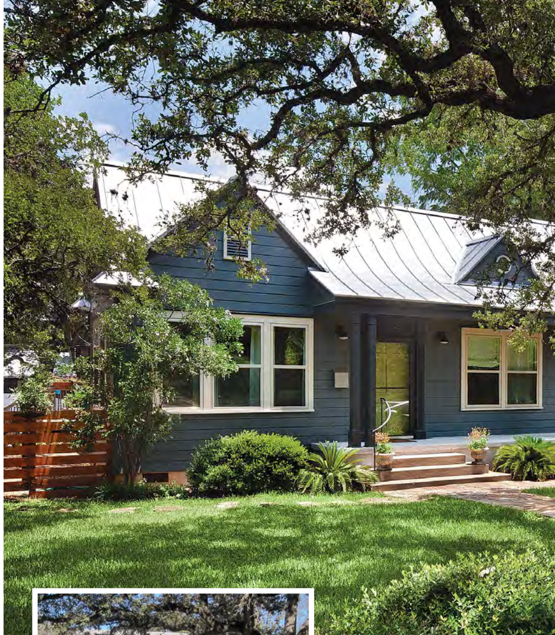
Expanding out and back. The front porch was completely rebuilt with a longer span. The new roof above the porch required special framing to match the curve of the existing roofline. Rafters were cut with a custom radius, and the metal roof was fitted to match.
