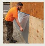
Overspray from the water-borne asphalt-based coating can stain concrete and masonry, so the first step is to cover those areas with painter's tape and plastic sheeting. The tape won't stick to concrete, so we apply it to the edge of the sheathing. The area under the tape gets coated with a brush later.
