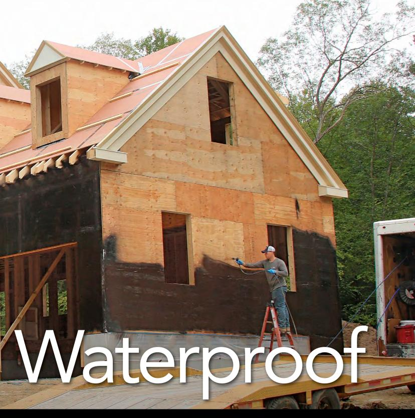
(12 perms) spray-applied water-resistive barrier (WRB) forms a continuous water-proof skin over the sheathing, greatly reducing air leakage and blocking water that gets through the siding. The asphalt-based coating will not blow off, it covers the sheathing nails to prevent water from following the nail holes into the framing, and it can be left exposed for up to 120 days. Although the sys-
