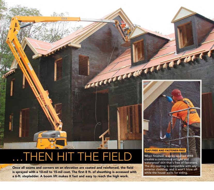
to shed water. We start with the horizontal and vertical seams on the first two rows of sheathing, and save inside and outside corners until the flat seams have had a chance to set up, usually about 15 to 30 minutes later. If we don't wait, the pressure from the sprayer can lift the joint fabric from the flat seams when we apply the coating to the corners.
