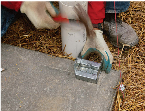
Locate post bases. Plumbing down from the rim, I mark and drill holes for the post-base anchor bolts, then install the bases. With the post ends wrapped in isolation membrane, I set the posts in place.
