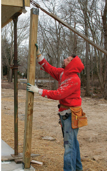
Locate post bases. Plumbing down from the rim, I mark and drill holes for the post-base anchor bolts, then install the bases. With the post ends wrapped in isolation membrane, I set the posts in place.
