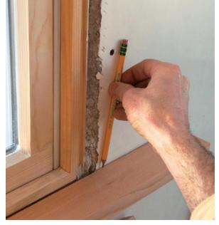
**Scribe the stool to the drywall.** Hold the stool in place, and with a pencil, scribe the profile of the wall onto the stool. I use a pencil for most scribing work, but you can also use a set of scribes or a compass.
