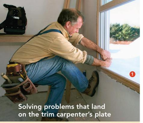
Built-up compound, loose drywall, bulges in framing, and poor window installations are some reasons the window jamb and the drywall might not line up. Like it or not, these problems become the trim carpenter's headache. If the drywall surface and the jamb edges aren't made flush with each other, you'll be fighting the trim through the rest of the project, and it might never look right.
