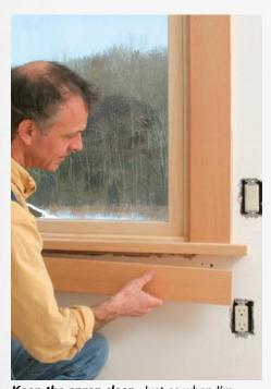
Keep the apron clean. Just as when I'm installing the side casings and the header assembly, I nail the apron carefully. Nails are best driven in pairs. I align pairs of nails vertically on the apron and header, horizontally on side casings.
