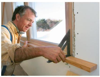
**Check for square.** While the stool is temporarily secured to the window jamb, check for square. The cause of any tilt should be eliminated to avoid a visible gap between the stool and the side casing.
