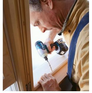
**Hide the fasteners if possible.** If the window molding is substantial enough, I screw the stool in place from the outside. I drive one 2-in. trim-head screw to secure the stool temporarily. Later, I add one every 8 in. for a permanent connection.
