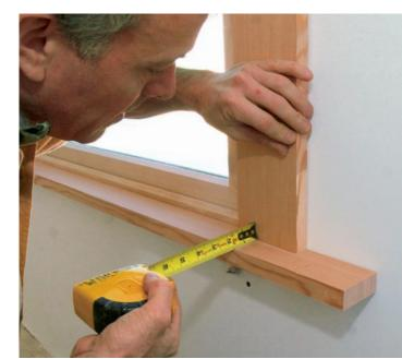
Size the stool in place. On the first window, I leave the stool horns long. With the stool temporarily attached, I hold the side casing in place and determine the stool length. A good rule of thumb is that the stool's side projection should match its front projection.
