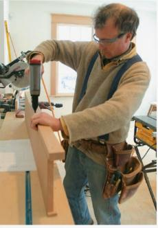
**Add a thin fillet and a fat cap.** Once the frieze is cut to length, I can nail the fillet along its bottom edge and the cap along the top. The thickness of the cap matches that of the stool.
