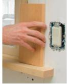
Move obstructions if necessary. I use a scrap of side casing to ensure that switch boxes and outlets aren't in the way. The box shown here is just far enough away that I don't need to call the electrician.
