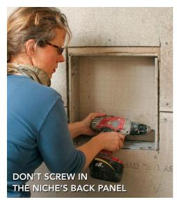
Measure, cut, and place a few beads of silicone caulk on the back of the niche's back panel prior to installing it. This piece is also held in place by the pressure of the niche's top and side pieces, which are secured with screws. TAPE ALL THE JOINTS AT ONCE
