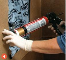
**CAULK SEALS BOTH MEMBRANES** I cut out the niche opening and seal the
