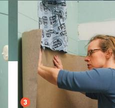
A VAPOR RETARDER KEEPS THE FRAMING AND WALLBOARD DRY I use Fortifiber's AquaBar (www.fortifiber.com), which is two layers of kraft paper laminated with asphalt. I attach it directly to the face of the greenboard or studs with staples, making sure to double-layer each corner for added protection. The bottom strip of niche flashing should lap over the vapor retarder.
