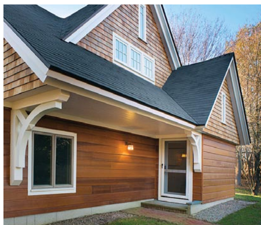
An inconspicuous front door becomes a subtle side entry. When the main entry was relocated to the west side of the house, the original entry became the side door it was meant to be. A robust bracket supports the deep overhang of the new roof. Photos taken at F on floor plan.
