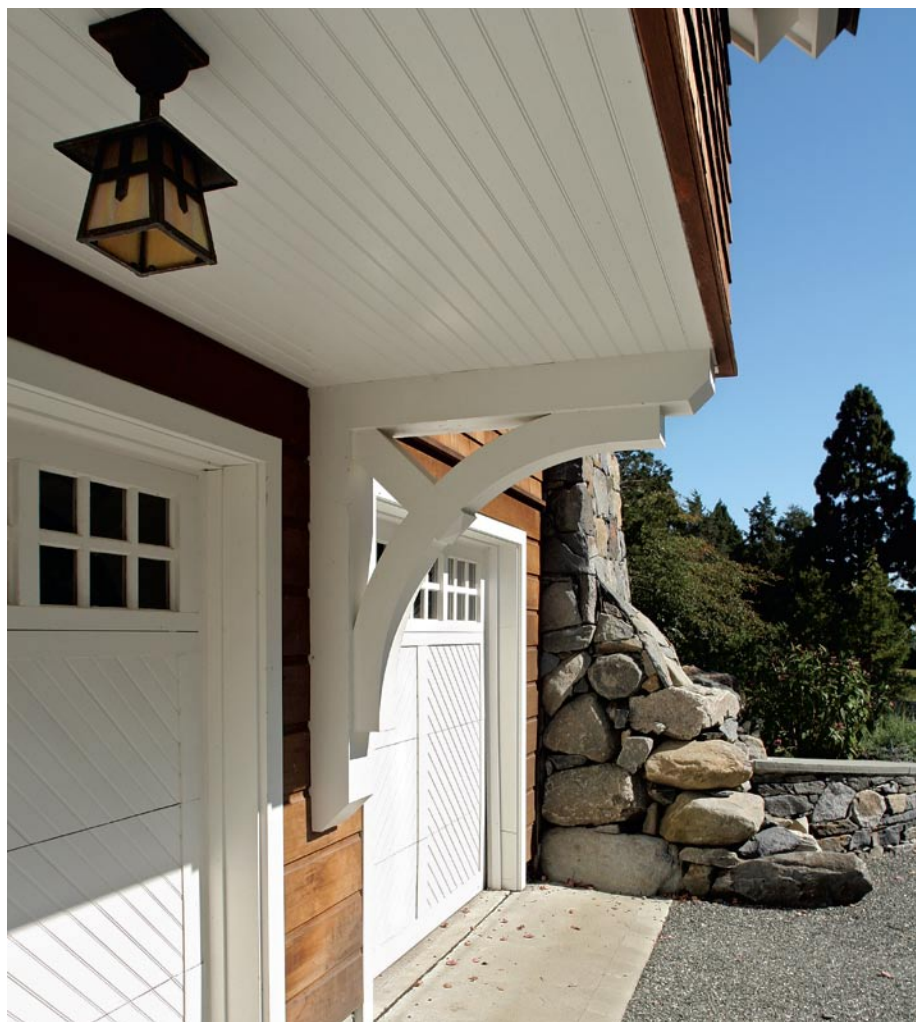
Boulders, brackets, and a place to park. Tucked away from street-front view, the three-car garage is treated with no less detail than the more-visible elevations. A cantilevered portion of the master bedroom shelters the garage and provides a place to mount lights. The chimney springs from the rubble of large boulders that project into the driveway. Photo taken at G on floor plan.
