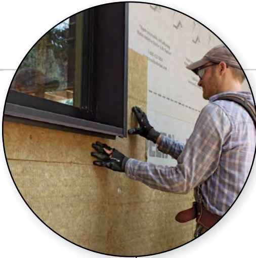
A warm jacket. Exterior insulation acts like a down coat to reduce the ability of framing members to transmit cold through walls. ComfortBoard 110 is dense enough to resist compression when the siding is attached.
