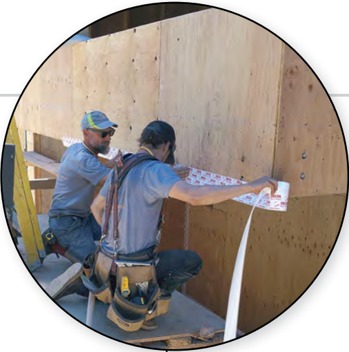
Exterior air barrier. The sheathing is air-sealed with Delta's self-adhesive, water-resistant air barrier. Wrapping the edges of the overhang first with Delta Multi-Band tape ensures a good seal.
