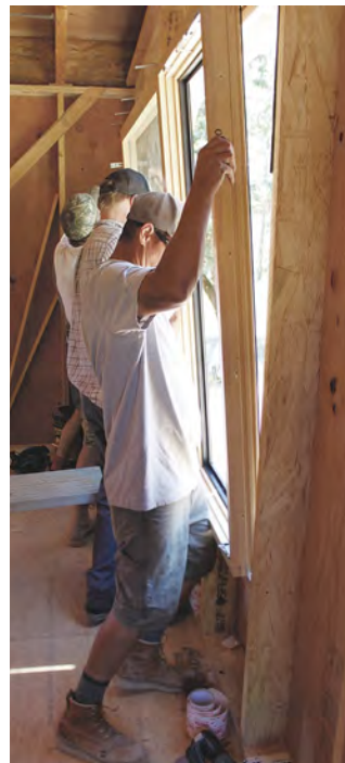
Securing the window. Zola windows are flangeless. Brackets are attached and the heavy window installed from the inside. 2x scraps tacked to the sheathing across each corner of the rough opening act as insurance against a dropped window. Screws through the brackets and the jambs secure the window.
