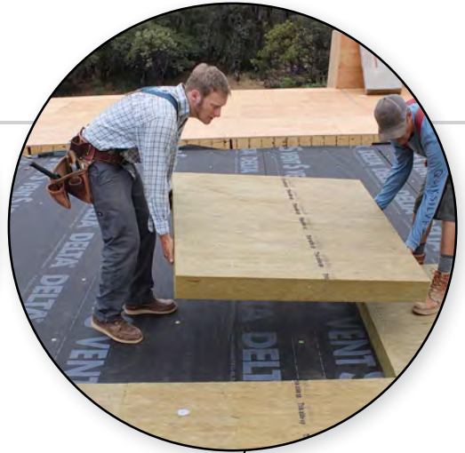
Moving the dew point. In this climate, 30% of the total insulation in an assembly should be on the exterior to prevent condensation on the sheathing. That's 5 in. of extremely dense Rockwool to support the standing-seam metal on a low-slope roof.
