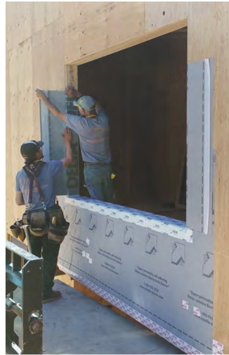
Start from the bottom. The peel-and-stick Delta-Vent SA wraps the opening. The self-adhesive WRB eliminates air leakage at the rough opening without additional tapes.
