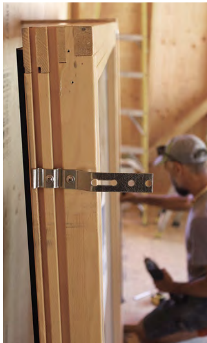
Securing the window. Zola windows are flangeless. Brackets are attached and the heavy window installed from the inside. 2x scraps tacked to the sheathing across each corner of the rough opening act as insurance against a dropped window. Screws through the brackets and the jambs secure the window.
