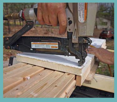
Vent baffles perform three tasks: they create an air gap between the insulation and roof, they prevent insulation from spilling into the soffit, and they provide an air barrier to minimize wind-washing of the insulation, which can compromise its R-value.
