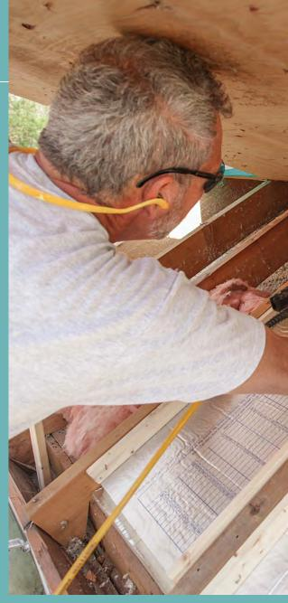
the baffles up the slope. The wood strips, meanwhile, act as spacers to keep the top of the baffles 15% in. or more beneath the roof sheathing, and also as a means to attach the baffles to the rafters.
