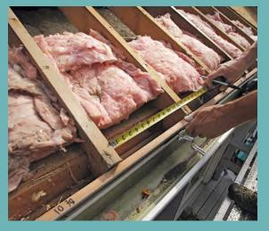
Foam and furring strips. Measure each rafter bay at the bottom and 4 ft. up, take the lesser of the two measurements—as long as they're less than ½ in. different—and write it on the fascia or top plate. If the measurements vary by more than ¼ in., you'll need a tapered baffle. On the ground, cut the 1-in. foam using a track saw, and attach wood strips on either side using ½-in.-crown by 1¾-in.-leg staples.
