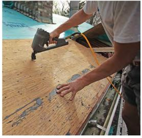
Punch them through. Specialty nail-removal tools are available, but you can also make your own by grinding the nose of an old framing nailer, allowing it to punch the sheathing nails through the sheathing to release each sheet from the rafters. We ground 3/8 in. of metal from the nailer's nose, and the driver (which strikes the nail) now projects 5/8 in.
