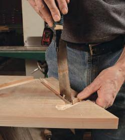
**Finish with a handsaw.** Use a handsaw to finish off the level and plumb cuts at the top of the stringers.
