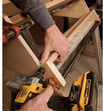
The rear portion of the landing tread sits on the subfloor, and is rabbeted the thickness of the finish flooring to sit flush with it. The landing tread doesn't get wedges. Instead, run small beads of glue in the mortises, drill countersunk pilot holes through the stringers and into the landing tread, and fasten with screws.
