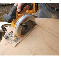
**Cut cleanly.** Clamp the template to sawhorses or a sacrificial base, and use a circular saw to make the long cuts for the risers and treads. Don't overcut; stop at the ends of the lines.
