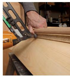
**Apply the cove.** Turn the stairs right-side up. Cut strips of cove molding to length, and attach them beneath the nosings with 1<sup>1</sup>/<sub>4</sub>-in. finish nails.
