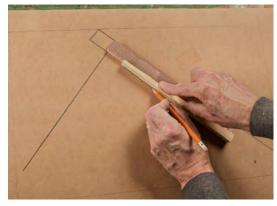
Lay out the template. Mark a 90° corner to start, extend a box out for the nosing, then use scraps of tread and riser stock along with precut wedges to precisely match the template's taper to the wedges' slope.
