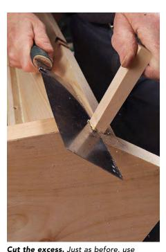
a handsaw and chisel to trim the riser wedges flush with or a bit below the stringers.
