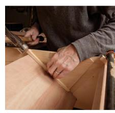
**Drive it home.** Insert the glued wedge into the mortise, and hammer it home with a few quick taps. Repeat the process with the topmost full tread and check for square. On long stairs, set a center tread next, then fill in the rest.
