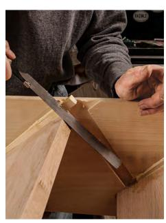
**Trim to length.** Use a handsaw to trim the long back ends of the wedges flush with the backs of the treads.
