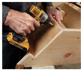
Like the landing tread, the topmost riser doesn't get wedges. Apply beads of glue to the back of the lower tread and under the landing tread, and insert the riser. Then drive multipurpose screws through the back of the riser into the stringer and into the back of the lower tread.
