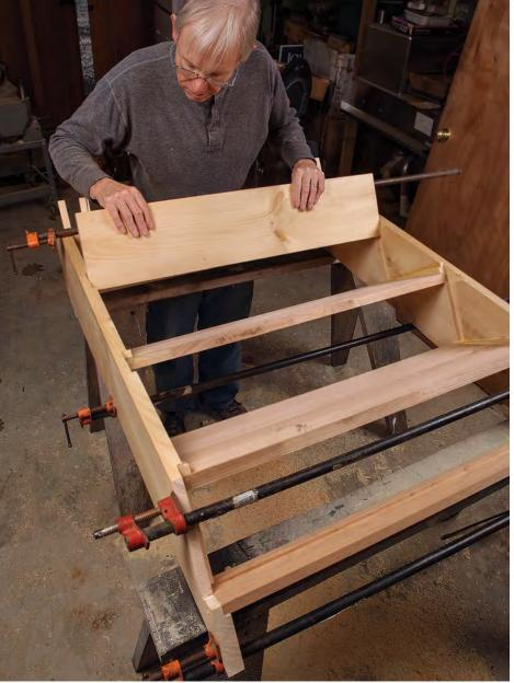
One at a time. If the risers are crowned, set them crown-up to match the bow of the treads. The intermediate risers are all the same height as the stairriser dimension. The bottom riser is one tread thickness shorter, and the top riser is typically <sup>1</sup>/<sub>4</sub> in. taller to tuck into the rabbet in the landing tread.
