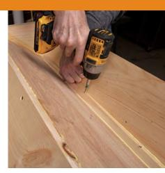
Reinforce the joint. Cut <sup>3</sup>/<sub>4</sub>-in.-square strips to length and glue and screw them in place to reinforce the back of the joint where the tops of the risers and the bottoms of the treads meet. Angle the 1<sup>1</sup>/<sub>2</sub>-in. screws slightly toward the tread nosings to pull it all tight.
