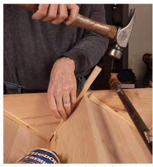
Wedge it. Using the same method as before, apply glue to the risers and wedges, and drive them home.
