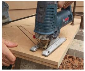
**Finish with a jigsaw.** Use a jigsaw to finish the cuts, and to cut out the nosing. Use sharp blades and a steady hand, as the router will follow any errors in the template.
