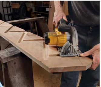
**Cut tops and bottoms.** Use a circular saw to make the bottom plumb and level cuts, and to start the plumb and level cuts at the top of the stringers. Don't overcut.
