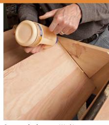
Start at the bottom. Working one side of each tread at a time, apply a bead of glue to the bottom of the tread, inside or just to the edge of its mortise. Run a similar bead of glue in the wedge where it will contact the mortise.
