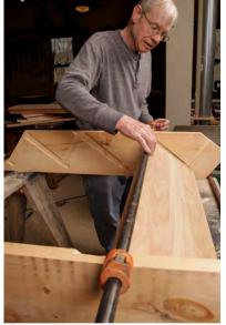
Stand it up. Stand the stringers backside-up about a tread's width apart on evenly matched sawhorses set on a flat floor. If the treads are bowed, orient the arches up. Fit the bottom tread and topmost full tread in their mortises, and clamp the stringers together top and bottom.
