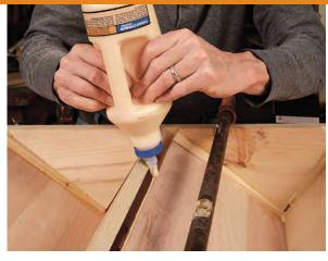
Glue the joint. Before wedging the risers, pull them back from the tread and apply a thin bead of glue to the back of the tread. Immediately allow the riser to fall back to the tread to spread the glue and prevent it from dripping onto the tread.
