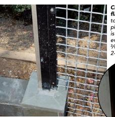
Clamp on the steel mesh with flanges. One flange is welded to the tubing. The other flange pinches the steel mesh fast and is fastened with bolts installed every 16 in. The steel mesh is <sup>3</sup>/<sub>16</sub>-in. stainless-steel wire on a 2-in. grid.
