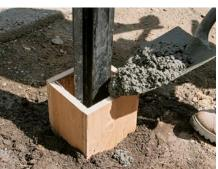
Make the base shed water. Simple forms made from scrap material work just fine for a small amount of concrete. After the concrete set up, the forms were removed, and a bluestone veneer was applied over the concrete (photo below). The tops were pitched so that water can't pool around the steel posts.
