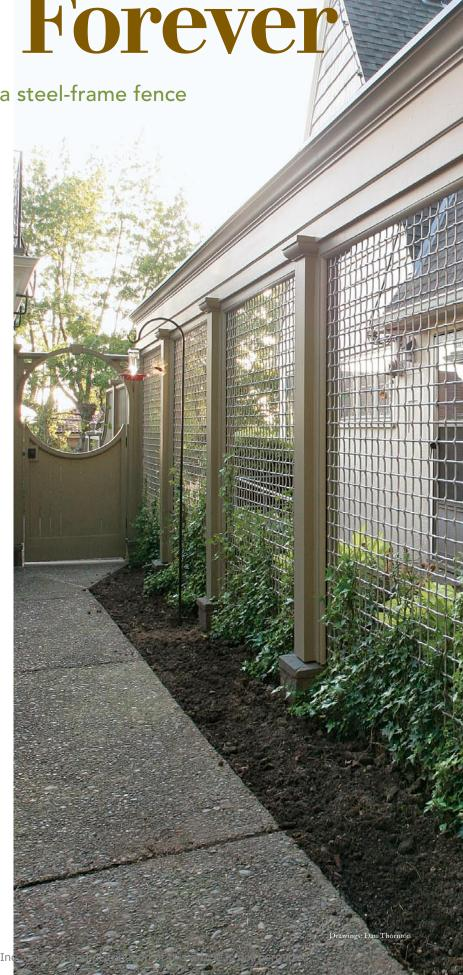
Set steel posts precisely with line, level, and spacers. When aligning a long run of posts, I leave nothing to chance. I always set the corner and end posts first. Once they're solidly anchored in poured
