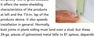
24-ga. pieces of galvanized metal (60¢ to \$1 apiece, depending on size) hold the ends of two abutting planks securely in place. Besides saving you the trouble of marking and cutting planks to land on a stud, and risking splits in the material by nailing so close to the plank edges, the off-stud jointer saves you from having to haul a pile of cutoffs to the landfill. Not bad results from a product that leaves only a small piece of painted metal at the bottom of the plank.
