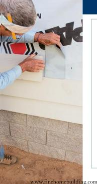
The off-stud jointer from Simplicity Tool is great because it offers the water-shedding characteristics of the products at left and the 11/4-in. lap of the products above. It also speeds
