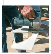
aggressive blade designed for use on fiberglass, cementboard, and fiber-cement products. Be sure to wear a respirator—or work in a Wyoming wind that will blow away the dust.
