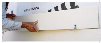
Malco has a metal gauge (\$21) that is designed to sit on the top edge of a plank. You can use either two metal gauges to hold and space the plank, or one metal gauge to hold the far end of a plank and an adjustable plastic spacer (\$10) to gauge the lap on the other end. Once the plank is nailed in place, the metal gauge is removed. Don't nail too close to the metal gauge, though, or it will be impossible to take out.
