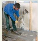
Take out only as much as you need. Scored by the sawcuts, the slab is easily broken out with a sledgehammer, then carted away in chunks.
