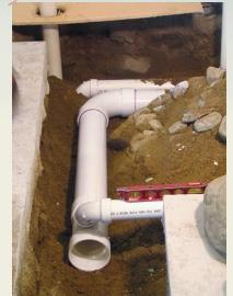
Keeping in pitch. As the plumber lays out the drains, he continually checks his work with a torpedo level equipped with a pitch vial.
