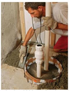
Isolate the tank lid, but not the tank. I use a ring of cardboard as a form around the sewage tank's lid so that the repoured patch sits on top of the tank rim but doesn't interfere with the removal of the lid. In some regions, seasonally high water tables can lift the tank right out of its hole if it's not secured.
