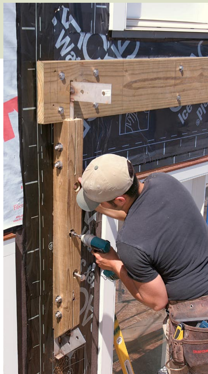
Framing members are cut to fit steel connectors. Sawkerfs are made with a circular saw, then cleaned out with a jigsaw so that the posts and ledger can slip over steel flanges and be bolted in place. The ledger and framing-connector posts are lag-screwed to solid-wall framing.
