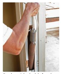
Put the weights back before the sashes. Because the weights I had weren't heavy enough, I added supplemental weights. The weights slip onto the sash cord and can be stacked on top of the main weights, as well as each other (2 lb. for \$12; www.architecturaliron.com). Once the weights are installed, I replace the access door to seal the side jamb.
