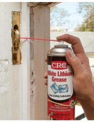
Lubricate the pulleys. Before reinstalling the ropes and weights, spray a lubricant into the housing onto the spindle/wheel center while you spin the wheel. Replace damaged pulleys with new ones. The one shown here from Van Dyke's Restorers (\$15.99; www.vandykes.com) includes nylon spindle bushings, which make for smooth operation.
