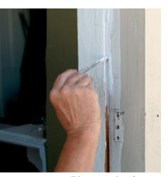
Prime all bare wood. Before reinstalling the sashes, I sand the jambs smooth, then prime and paint them to create a tough, slippery surface. I like DuPont's Corlar and Imron products, but they are available only through industrial suppliers. As an alternative, a high-gloss marine enamel works well.
