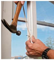
A knot and a finish nail do the trick. A knot at the end of the sash cord sits in a hole in the sash stile. For extra hold, I run a finish nail through the knot. I bend the remaining length of nail over the knot to push the knot into the channel so that it won't rub on the side jambs.
