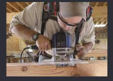
Although you could always use a chisel, I cut the notches where the beams rest on the posts using a slightly different approach. After knocking out the circularsaw waste, I flatten the bottom using a router mounted to an oversize base and armed with a bearing-guided bit.
