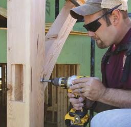
Clean holes. After fitting each angled brace, drill the holes for the 1-in.-dia. oak pegs that will hold them tight. Start each hole with a 1-in. Forstner bit, which leaves clean edges, and then switch to a heavy-duty auger bit for the bulk of the work. Stop the auger bit just shy of going all the way through, then switch back to the Forstner to finish the job from the opposite side.
