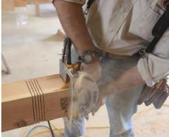
**Score with a circular saw.** After marking the shape of the tenon on the sides and end grain of the timber, use those marks to set the depth of cut on your circular saw. Then, score the waste to make it easier to knock loose.
