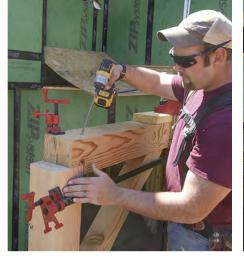
Fit the braces. After coercing the braces into their mortises, pull everything tightly together with a pair of clamps, and then secure the post-to-beam connection with long structural screws driven at an angle.
