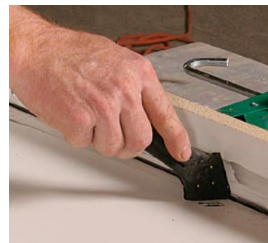
Clean fingertip, smooth bead. After applying the silicone with a caulk gun, spread it with a caulk tool.
