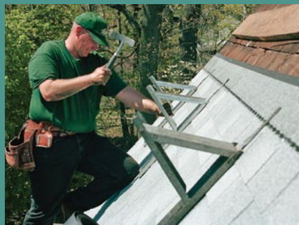
Slater's roof jacks are extrawide. This allows them to hold up to a 2x12 plank rather than a 2x10 typical of other roof brackets ($33 each at www.slate-roofcentral.com ).
