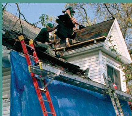
Catch the shingles. Roof jacks with a 2x12 catch the shingles while a scaffold below provides a place to stand and toss shingles into the landing zone.
