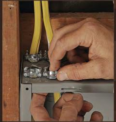
Work back to front. Box connectors secure cables and protect them from the knockouts' sharp edges. Start from the back; otherwise, the front cables will block access to the rear connector's set screws. Feed the cables in two at a time, and use cable stackers to keep them organized.
