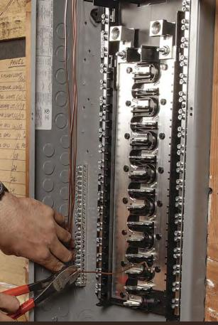
Work from the bottom up. Hold your finger on the wire across from the bus-bar location where you're going to attach it, make a soft 90° bend, and cut the wire to length. About ½ in. of copper should stick through the other side of the bus. Leave the bottommost space on each ground bus bar open for a jumper.
