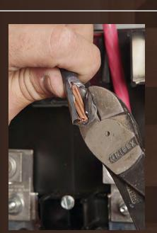
**Twist and split.** Use diagonal cutters to split and peel the insulation away from the feed cables.
