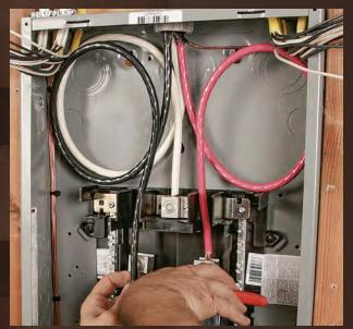
**Don't stress the subfeeds.** After connecting the neutral feed, move on to the hot-feed cables. Loop each cable once so its end goes square into its lug. Line the cable up with the lug to determine where to trim it, then cut at that mark with diagonal cutters.
