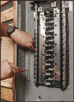
**Two is better than one.** Most panels come with one ground bus bar. To keep things neat, I install a second—one for each side of the box.
