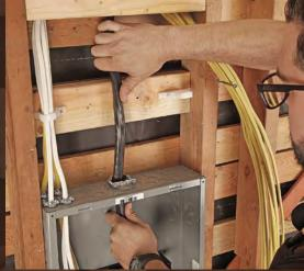
Erase the memory. The subfeed cable in particular is stiff and has a "memory," or tendency to return to its original shape, which can strain connections if it's not worked out. Take your time to get it as straight as possible before tightening the connector's set screws.
