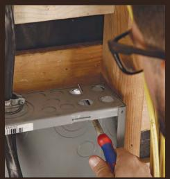
Tap and pull. To remove the metal knockouts, tap them down with needlenose pliers, and then pull them out from the bottom.
