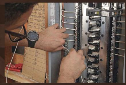
Neutrals come next. Land the neutrals in order from top to bottom. Push the wire to the back corner of the box, run your finger down it until you're even with the space on the neutral bus where it's going to land, hold your finger on the wire as a bending point, and bend a soft 90° with your other hand.
