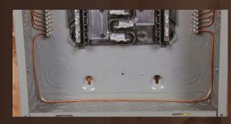
Ground connection. I connect the ground bus bars with the cutoff from the subfeed's ground wire. This connection isn't required, since the ground buses are connected to the box, but it's an extra measure that guarantees the grounds are tied together.
