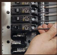
**Install the breakers.** With the breakers snapped into place, bend the hots, strip out ½ in. of insulation, and connect the hots to each, tightening the set screws.
