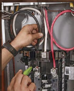
**Plug it in.** Insert the feed cables into the lugs, leaving about ½ in. of copper exposed at the top so you don't pinch the insulation. Zip-tie the service loops together so they stay neat.
