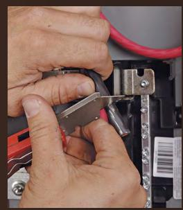
**Strip an inch.** Use a utility knife to score a line around the insulation of each feed cable.
