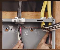
The last ground. Install an insulating bushing onto the connector holding the feed cables, then separate out the feed's ground wire, bend it to the right side of the box, connect it to the ground bus bar along with the other grounds, and zip-tie that group too.
