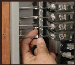
Label the hots. Although the temporary labels have been removed, I label the hots more permanently so the next person who opens the panel can easily identify which circuit is which.
