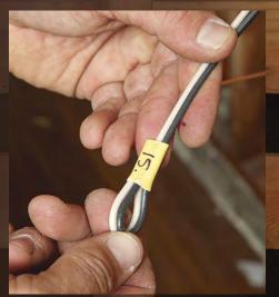
Reuse the label. Slip the label over the ends of the neutral and hot wires, bend the ends over, and secure the wires' tips under the label to hold it in place.
