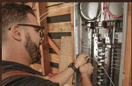
Cut, strip, tighten. Use wire strippers to cut off the excess, strip about ½ in. of insulation from the end, and insert the wire into the neutral bus bar just far enough that a little copper shows out the other side. You can always cut the wire a little long and nip it back. Zip-tie the neutrals together on either side of the box.
