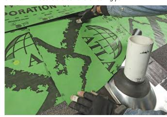
**Extra protection.** Cut and install a piece of underlayment that laps 6 in. beneath the next underlayment joint above, and down onto the top of the flashing boot's pan.
