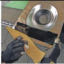
Dam the rain. Remove the backing on one half of the tape, then center and bond it to the underside of the bottom portion of the flashing pan. Then fold the flashing tape back on itself and remove the second strip of release sheet.
