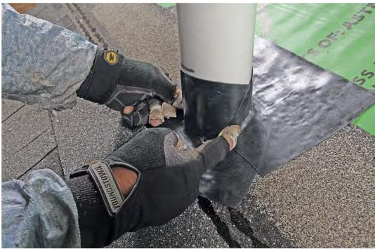
**Tape the upslope.** Using the same method as the downslope side, apply the second piece of tape so it overlaps the first around the pipe, again staying  $\frac{1}{2}$  in. below the collar mark.
