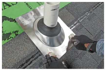
**Boot it.** With one hand under the pan holding the tape flap so the sticky side stays down, slide the flashing boot over the pipe, align the flashing pan square with the roof shingles, and press the bottom edge down to seal the tape.
