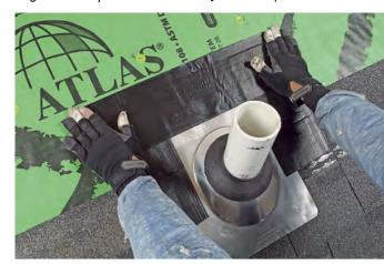
**Tape the head.** Cut a strip of 4-in. to 6-in. flashing tape long enough to cover across the tops of the side strips of flashing tape. Overlap the top of the pan flashing, keeping the bottom edge of the tape about ½ in. to 1 in. above the bell of the flashing pan.
