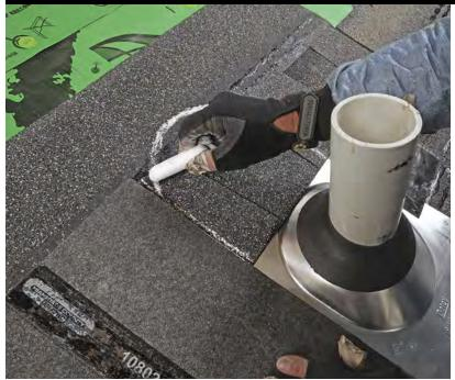
**Trim shingles to fit.** Continue shingling. When you get to the vent pipe, mark the cutout for the vent pipe on the shingle, using another shingle as a straightedge. I eyeball the curve around the flashing boot's bell.
