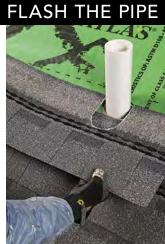
Shingle up to and around the pipe. The top edge of the last course of shingles to go on before the flashing tape should extend at least to the middle of the pipe, but no further up than the self-seal strip on the shingle. Hold the shingle in place below the pipe and mark the cutout with chalk.
