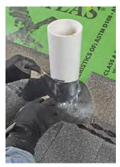
Tape the downslope. First, mark a line on the pipe representing the top of the vent boot's collar. Fold the tape in half lengthwise, with the adhesive side out, and, starting from the middle and ½ in. below the mark, wrap the tape around the pipe, working one side at a time.
