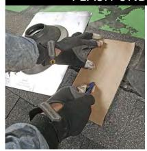
**Score the backing.** Cut a piece of asphalt flashing tape about 1 in. narrower than the width of the flashing pan, and use a utility knife to score the release sheet down the middle so it can be removed in two steps.
