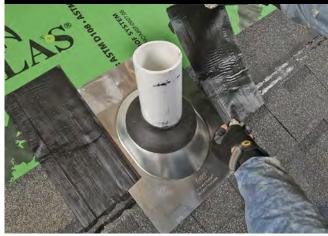
**Tape the sides.** Cut two strips of 4-in.- to 6-in.-wide asphalt flashing tape and apply it over the sides of the flashing pan and onto the shingle and underlayment. Keep the tape above the shingle's self-seal strip, and let it extend 1 in. to 2 in. above the pan. Keep the edge of the tape about ½ in. away from the pan's bell.
