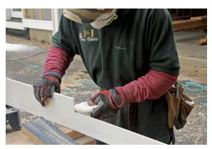
**Prime cuts.** Cut ends, even in fiber-cement siding, will wick moisture and lead to degradation and peeling paint. We prefer to apply primer with a foamtipped squeeze bottle, much like a liquid shoe polish.
