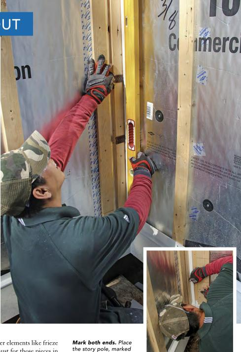
Mark both ends. Place the story pole, marked with a 4-in. siding exposure, on top of a 1/4-in. shim that creates the manufacturer-required gap above the water table. Once in place, transfer the siding courses from the story pole to the furring strips at both ends of each run. Snap chalklines between the marks so the siding can be easily aligned for its entire length.
