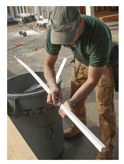
**Ease the back.** Chamfer the hidden edge of the inside-corner stock with a block plane before installation to ensure the 1-in.-square stock will sit tight to the underlying furring strips.
