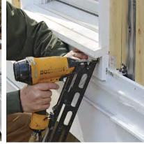
Windows wear an apron. Cut the 5/4 PVC window aprons with a bevel at the top that matches the slope of the sill and a notch on the back that matches the angle of the lap siding. The size of the notch varies with the layout of the courses, so each is custom-cut.
