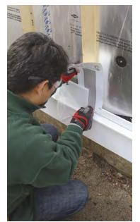
Flash butt joints. Cut siding planks so that any butt joints land in the center of a furring strip where they can be backed up with flashing (bearclip.com) before being nailed about ½ in. from the end of the plank. Offset seams at least 2 ft. and arrange them so they don't create a repeating pattern.
