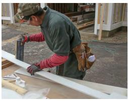
**Clean up corners.** Instead of overcutting the corners, stop the vertical cuts of a U-shaped cutout at the layout marks on the panel's front side. Then break off the waste piece and square up the corners with a utility knife.
