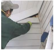
**Frieze overlaps siding.** The final course of siding at eaves and gable ends is pretty forgiving to install thanks to the packed-out frieze, which allows pieces to be slipped into place.
