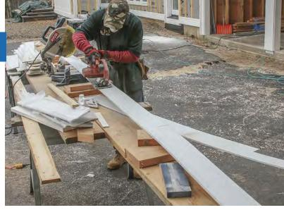
**Work around windows and doors.** The tops and bottoms of windows and the tops of doors often require a U-shaped cut. We prefer to make these cuts using a circular saw equipped with a fiber-cement blade.
