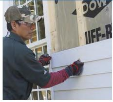
**Shim for an even gap.** When measuring and fitting each plank, use an ½-in.-thick shim at either end to ensure a consistent gap where the ends of siding planks butt into trim boards.
