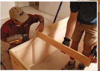
Attach the top panel and head jamb. Using the length of the original head jamb as a guide, I screw the top panel and nail the original head jamb to the side panels. I ripped <sup>3</sup>/<sub>4</sub> in. off the original head jamb so that the filler panel will tuck in front of it once it's installed.
