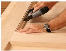
Add plywood and panel molding. After gluing and nailing %4-in. birch plywood to the back of the panel frame, I use a headless pinner to apply the poplar panel molding. All the vestibule panels are built the same way.
