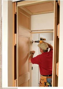
Install the hinges, then hang the door. Once the hinge side of the jamb is nailed plumb, I install the hinges. Whether I'm hanging a hollow- or solid-core door, I run a long wood screw through the middle hole of each hinge to catch the framing by at least 1 in. I then shim and nail the other side jamb in place, maintaining an even reveal around the door once it's closed.
