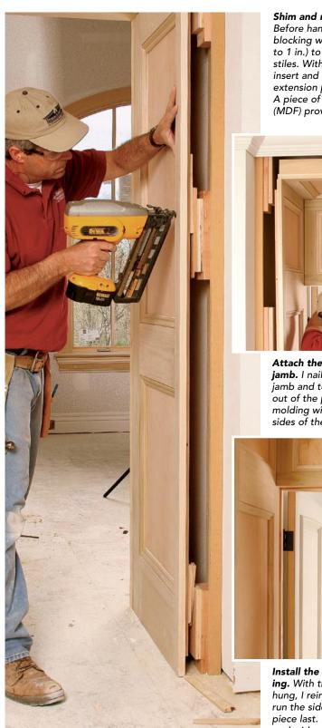
Shim and nail the outer stiles plumb. Before hanging the unit, I installed blocking within shimming range (½ in. to 1 in.) to sit behind the extension's stiles. With the door jamb nailed off, I insert and adjust shims to get the jamb extension plumb before nailing it off. A piece of medium-density fiberboard (MDF) provides backing for the casing.
