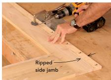
Join the jamb to the assembled frame. I assemble each extension's frame with pocket screws. Once all the frames are built, I join the ripped side jamb to the frame of the extension with glue and pocket screws spaced every 6 in. When the unit is assembled and the door is hung, I reattach the doorstop over this joint.
