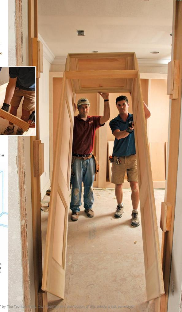
Shim the jamb plumb, then tack it in place. I plumb the hinge side of the unit first, then nail it in place with 2½-in. trim nails. I keep these nails in the area of the jamb that will be covered by the doorstop so that there are fewer holes to fill later.
