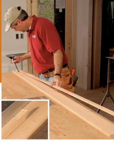
Remove the doorstop molding, then rip each side jamb. After disassembling the jamb, I pry off the doorstop carefully so that it can be reinstalled later. I rip the side jamb down to 2 in. I also rip ¾ in. off the head jamb so that the filler panel will tuck in front of the head jamb when the unit is installed later.
