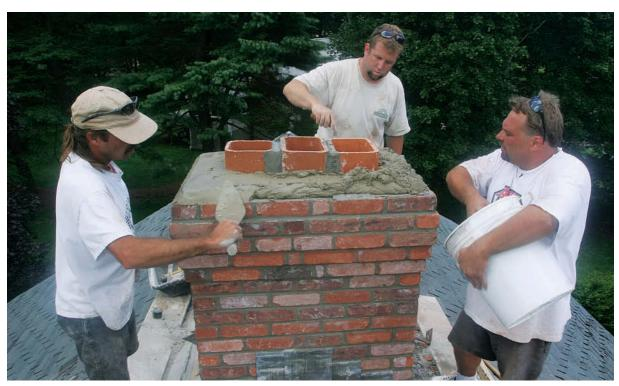
Masons finish up a repair on a three-flue chimney. In airtight houses, chimney flues often offer the path of least resistance for makeup air for combustion appliances and range hoods, leading to a sooty smell inside the home.
