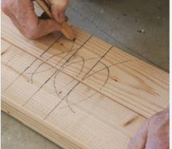
X marks the spot. Every standard-height stud is marked on the plates with an X. With the two plates next to each other, you can quickly mark an X on each by making two Cs, one backward.
