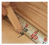
Regular studs follow a regular layout. The highlighted numbers on the tape—usually in red—indicate the common 16-in.-on-center spacing, but layout requires the edges be marked, not the centers. To mark the edge of a 1½-in. stud, subtract <sup>3</sup>/<sub>4</sub> in., and mark an X to the right.
