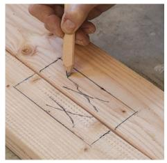
Be careful at intersections. Mark both edges of midplate wall intersections. For intersecting 2x4 walls, mark the plates to receive a 2x6 on the flat. The wider stud will extend past each side of the intersecting 2x4 to provide drywall nailing.
