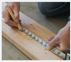
Mark the point loads first. With the plates laid next to each other, mark the edge of all the studs in point-load posts using dimensions from the blueprints.
