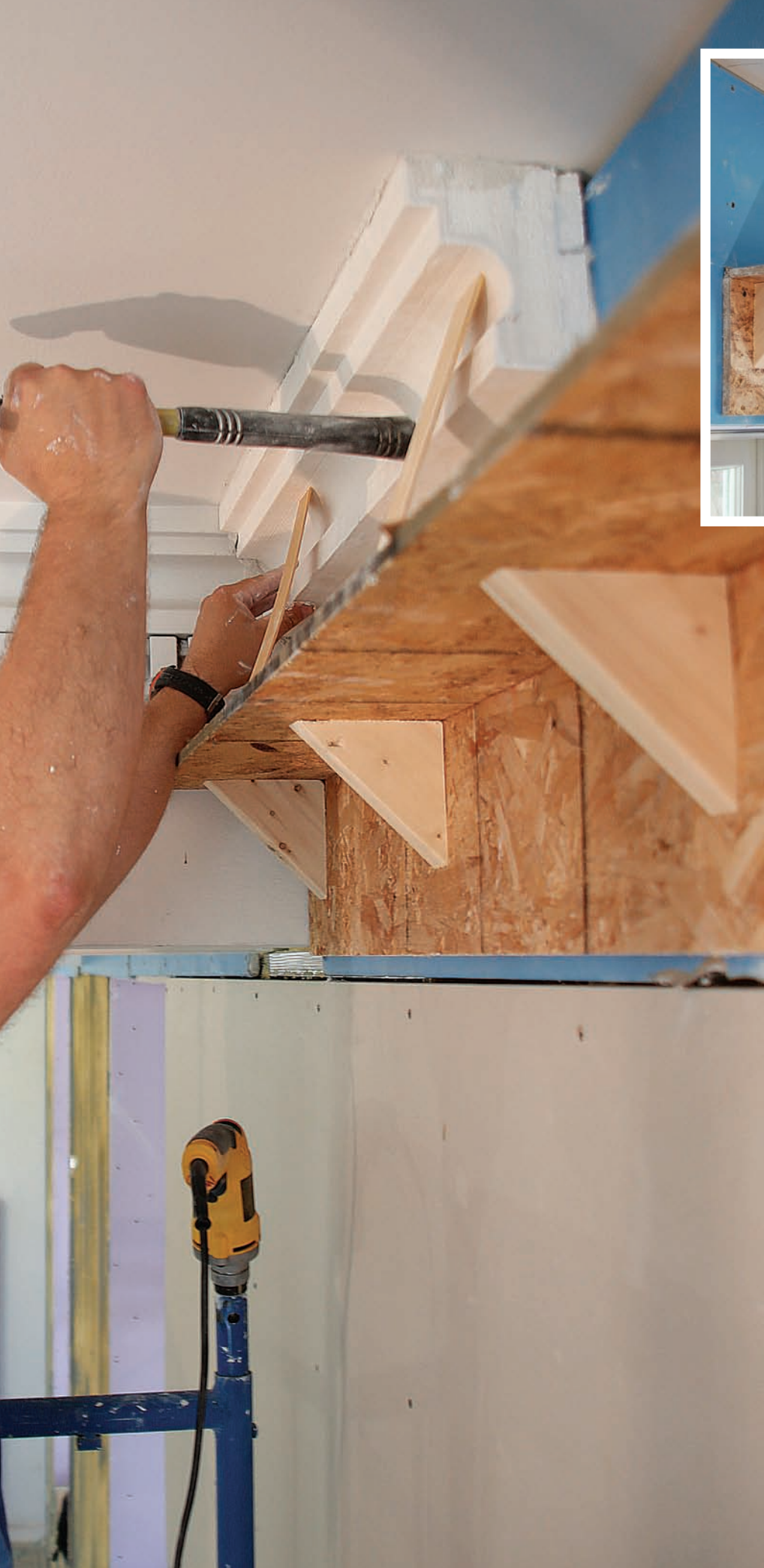
Butter the butt joints. Use a trowel to spread base-coat plaster onto molding edges when joining pieces for a long run.
