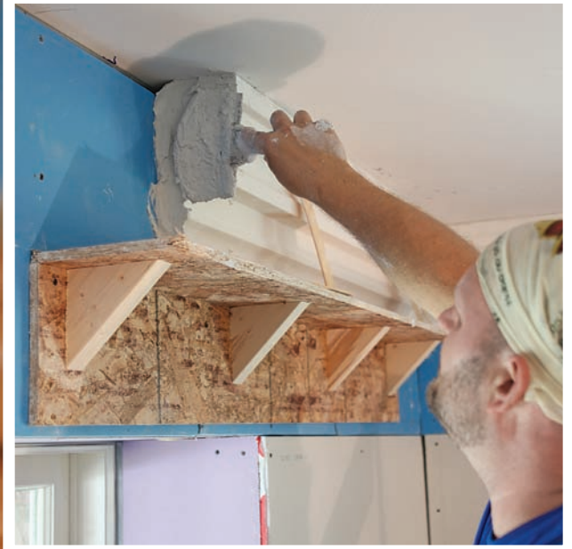
Butter the butt joints. Use a trowel to spread base-coat plaster onto molding edges when joining pieces for a long run.
