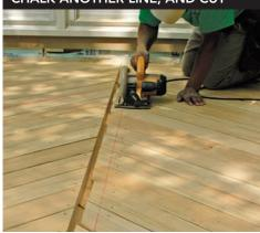
**Trim the centerline.** Once the decking is installed, snap and cut a line on the parting beam to create the exact space for the parting board that will run down the center. A straight line looks better, so work slowly, follow a guide, or use a track saw.
