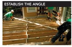
Run the first board from the corner. The 45° decking angle is established by measuring a right triangle from the intersection of the house and the parting beam, then snapping a chalkline as a reference for the first board.
