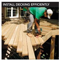
Cover the area quickly. For better workflow, lay out the decking from the first board toward the perimeter, leave it long, and tack it into position. Later, go back, drive all the remaining screws, and trim the board ends where they overhang the perimeter.
