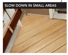
This is the place for precise cuts. Once the outer portion is filled in, the inner corner can be tackled. Hemmed in by the house, each board must be cut to fit on both ends.
