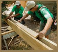
A parting beam, added during the framing stage, supports the board ends at the center of the deck. Join two joists with a full-length 2x4 along the top edge and 2x4 blocking underneath.
