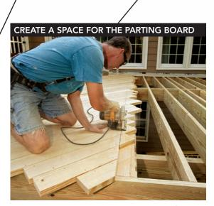
Chalk the midline, and cut. When one side of the decking is complete, chalk a line just inside the parting beam, and trim the deck-board ends at the line. Always use blue or white chalk; red is indelible.
