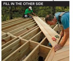
**Start in the middle.** To establish the duplicate angle, dry-lay a group of three boards, aligning them with the opposite side. Starting in the middle reduces the chance of accumulated error. Check the angle, then fasten the boards and fill in on both sides of the group.
