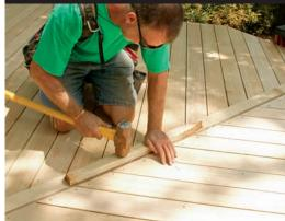
**Make it tight.** Rip the parting board with a slight bevel on both edges so that it fits snugly in the space between the two fields of decking. A sledgehammer and a block help persuade the fit.
