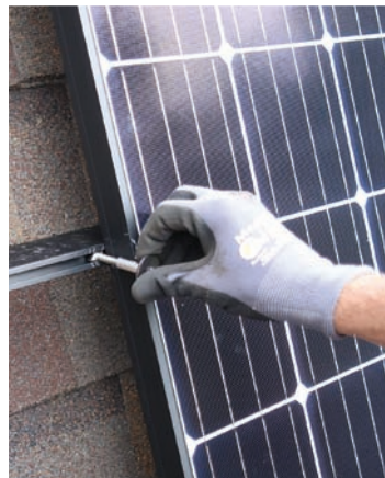
Shared fasteners. Mating modules are clamped to the rails with a shared T-bolt that is part of the mounting system.
