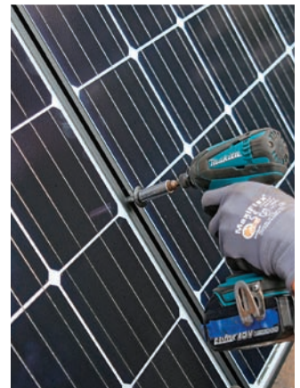
Shared fasteners. Mating modules are clamped to the rails with a shared T-bolt that is part of the mounting system.
