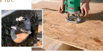
Cut openings quickly with a panel-cutting bit. I look for a plunge-cutting panel bit with a cutting length of 11/8 in. or 11/4 in. This allows me to get twice the life out of the bit: After I dull the top half, I reset the bit lower for a fresh cutting surface. Porter-Cable makes one for around \$16.
