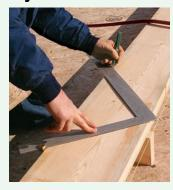
With stair buttons attached to the tongue and blade of a framing square, you can mark the gable wall's stud layout right on the face of each rafter. Button position depends on roof pitch. The 1½-in.-wide tongue of the square should remain perpendicular to the wall's bottom plate as you move up the rafter, stepping off a 16-in. run. Tracing against the edges of the tongue gives you the placement of the stud.
