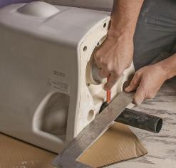
Fit the inlet and outlet pipes. Both the inlet and outlet pipes are measured in the same way. First, lubricate the pipe with soapy water and fully insert it into the carrier. Mark the wall location onto the pipe using a sharp pencil and a straightedge. Remove the pipe from the carrier and fully insert it into the opening at the back of the bowl, then mark how far it enters the bowl. Measure between the marks and add  $\frac{1}{8}$  in. Cut this amount from the end.
