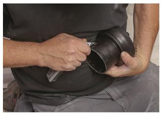
**Chamfer the ends.** After cutting the parts to length, use a knife to remove any burrs and then chamfer the cut edges with a file. This important step prevents damage to the O-rings that seal the pipe connections as the parts come together.
