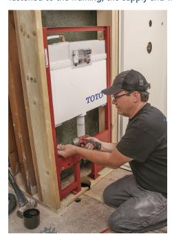
Fasten the carrier. The carrier, which is rated to support 880 lb., is secured to the framing with eight lag screws driven into predrilled holes. Six screws go through the sides of the frame and two fasten the legs to the bottom plate.
