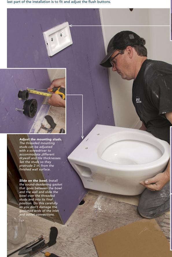
Set the depth. Adjust the clear-plastic access panel behind the flush buttons so it's inset ½ in. from the finished wall surface. Removing the clear panel provides access to the shutoff and all of the tank's internal parts so they can be serviced or replaced.
