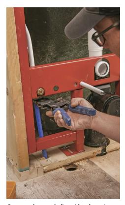
**Connect the supply line.** After fastening the carrier, connect the supply line. Because the connection will be hidden behind the drywall, the shutoff valve is remotely located behind the panel that houses the flush buttons.
