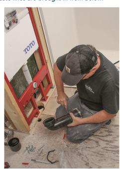
**Prepare the waste line.** The kit includes a 3-in. elbow that fits within a 2x6 wall. A flexible coupling attaches the elbow to the waste line running below the floor. The elbow is snapped into place and held in position on the carrier with a U-shaped plastic clip.
