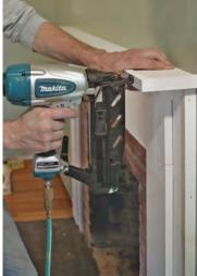
A stronger shelf. The MDF mantel shelf is likely to take abuse, and therefore demands a hardwood nosing. To ensure alignment and help provide positive fastening, use a tablesaw to cut both shelf and nosing with nesting rabbets, leaving a slight reveal on the top and bottom to create a nice shadowline and eliminate the need for sanding in place.
