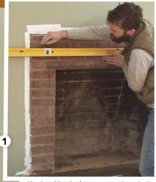
**Plumb and level.** After measuring the setback from the edge of the firebox to where the inside edge of the foundation boards will land, use a pencil to strike dead-level and plumb lines across the masonry.
