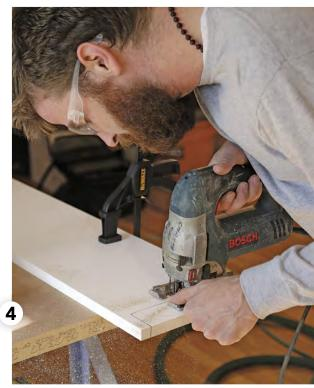
**Beveled for a tight fit.** Cut along the scribed line using a jigsaw set to a slight undercutting bevel, taking the back edge of the board out of the equation to ensure the front sits tight to the hearth.
