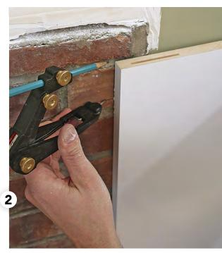
**Get set to scribe.** After aligning the inside edge of each vertical foundation board to its plumb line, set your scribes to equal the distance from the top of the board—which is left longer than necessary—to the level pencil line on the masonry.
