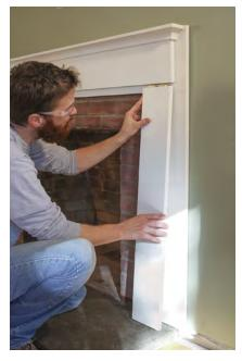
In and up. Left just short of full length to allow for an easy fit, each pilaster gets glue and biscuits along the top edge before being slid up tight to the underside of the frieze. The gap at the bottom will be covered by the base detail.
