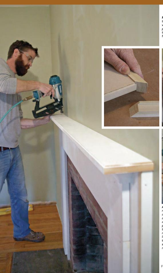
Hide the top. After scribing the mantel shelf to fit any waves in the wall, set it in place and fasten it down to the frieze assembly with finish nails.
