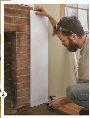
Mark the bottom. Still holding the extralong foundation board in position, trace the contours of the hearth onto the bottom face of the board. Once cut away, the board will fit at the bottom and be in alignment at the top.
