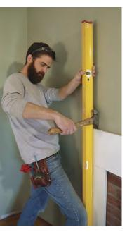
Pry it plumb. Once the glue sets, the foundation boards will act as a single unit. At this point, it can be pulled away from the wall as much as necessary to get it plumb before adding a few more finish nails through and into the framing around the masonry.
