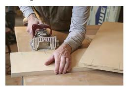
Biscuits for alignment. The three pieces that make up the foundation assembly are joined together in place rather than installed as one piece. To ensure flush joints that stay tight, the parts are slotted for biscuits and gluesized before installation.
