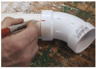
Make your marks. When joining fittings such as elbows or tees in a place where orientation matters, dry-fit the parts and make alignment marks on the pipe and the fitting.
