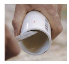
**Sevel the inside.** With the round side of the file, chamfer the inside of the pipe.
