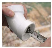
Find the fitting depth. Measure to the ridge inside the fitting to find how much pipe to allow for the joint.
