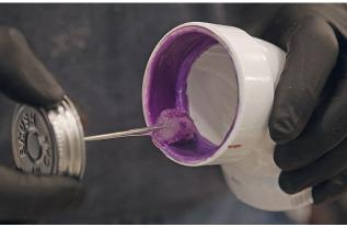
Cement the fitting. Without rewetting the applicator, apply a light coat of cement inside the fitting, then apply a second coat of cement to the outside of the pipe.
