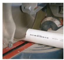
**2** Cut the pipe. A miter saw with a regular blade does a good job making clean, square cuts.
