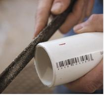
Bevel the outside. Use the flat side of a mill bastard file to create a 45° chamfer on the pipe's end.
