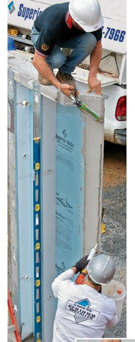
All joints are sealed with urethane. Corner panels are mitered; the others butt together. The crew uses Bostik Chem-Calk Smooth Urethane Sealant (www .bostik-us.com) on all panel joints before bolting them together.
