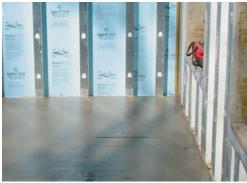
A concrete slab anchors the bottom of the walls. To brace the walls before backfilling, a slab is poured inside the walls; the floor framing secures the top. A pressure-treated 1x4 fastened around the inside perimeter acts as a screed and keeps concrete out of the wall cavities.
