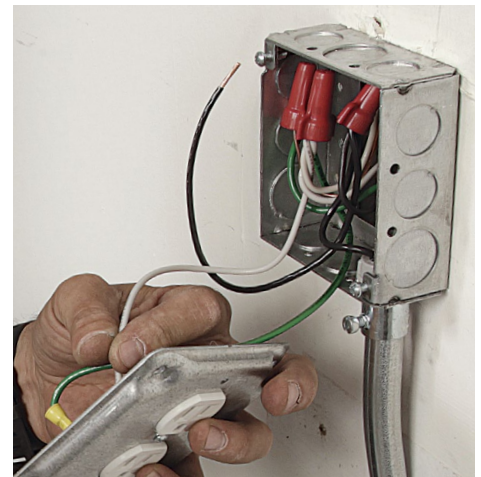
Mount devices. Devices installed in surface-mounted boxes are attached to the faceplate rather than the box. Break the ears off the device with pliers and attach the cover to the device with the provided screws.
