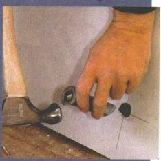
Once their centers are laid out, plumbing supply lines and other small protrusions are quickly punched out with a scrap of <sup>3</sup>/<sub>4</sub>-in. conduit.
