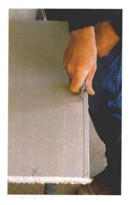
**One-handed rip guide.** For narrow rips, the thumb on the cutting hand serves as the rip guide. Because it's difficult to remove a narrow piece without damage, the backside must be scored as well as the front.
