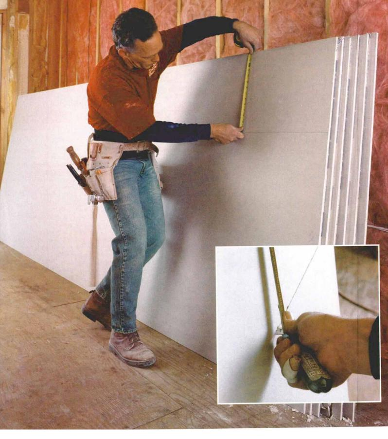
**The way the pros rip drywall.** To make his tape measure serve as a makeshift rip fence, the author pushes the hook on the end of the tape against the knife blade that he holds in his right hand. With his left hand, he pinches the tape between his thumb and index finger; the index finger serves as the fence that runs along the factory edge of the board.
