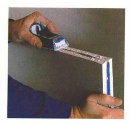
Two for the price of one. After cutting a sheet but before separating the two halves, the author makes one pass with a Surform pocket plane to smooth the rough spots on both edges at the same time.
