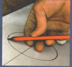
Rotating a pencil around a drywall nail that's gripped between thumb and forefinger works like a compass for drawing large circular cutouts.
