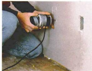
A perfect box every time. Rather than measuring, marking and sawing, a router makes errorproof cutouts after the board is in place. Predrawn arrows on the floor designate the center of each electrical box.
