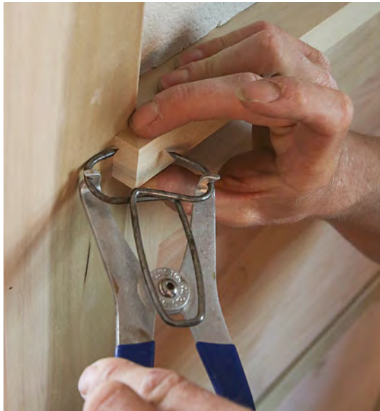
Glued returns. Extend the cap over the casing edges, mitering the very ends. Cut small returns and glue and clamp them into place.
