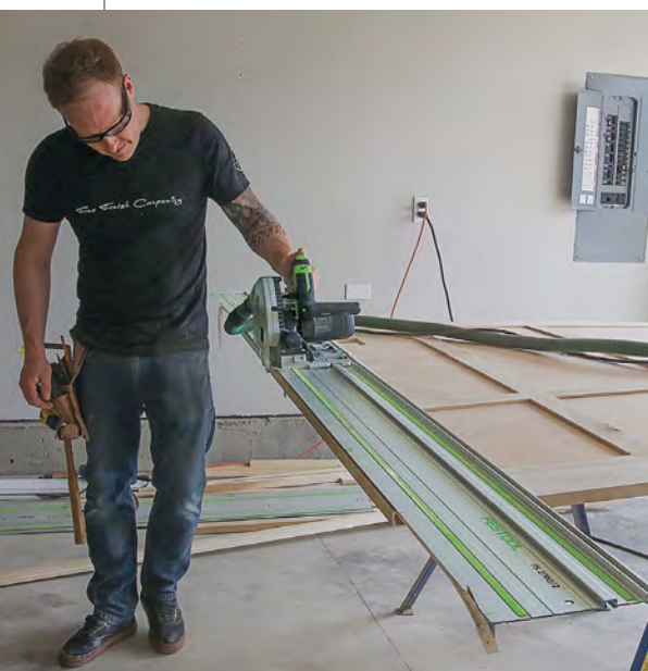
Trim to fit. Make the panels a little oversize in the shop, then cut them to size on site. A track saw is a great way to make the finish-grade cuts required for final fitting.
