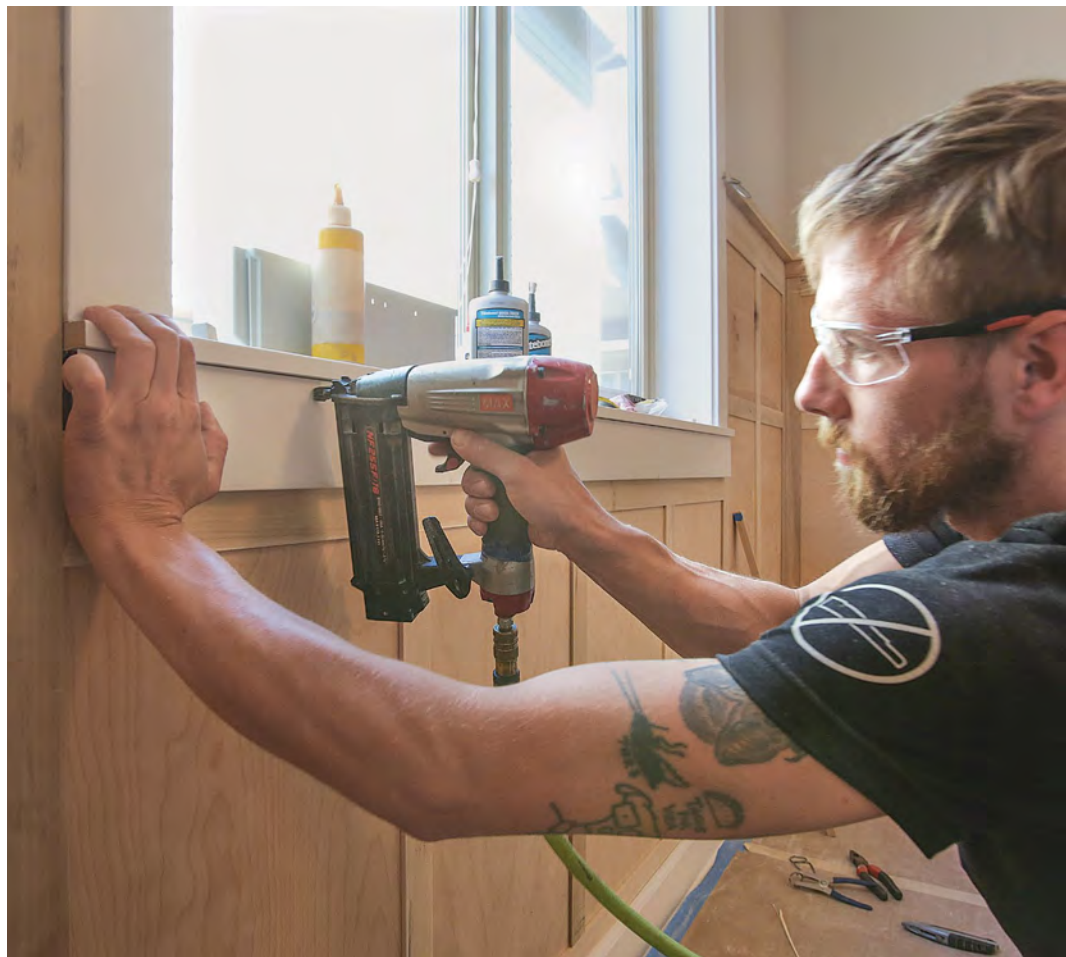
Reinstall the old trim. Retaining the existing molding profiles around common details such as windows and doors visually ties the new wainscot to the rest of the house.
