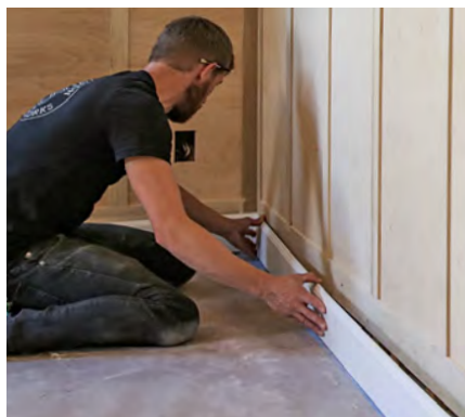
Flex fit. Cut base molding a little long so that it meets the perpendicular piece in a cope and snaps into place.
