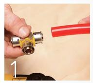
Slide the fitting onto the tubing.
