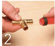
Align the crimp ring so that it's about <sup>1</sup>/<sub>8</sub> in. to <sup>1</sup>/<sub>4</sub> in. from the end of the tubing. Aim to have the ring aligned over the fitting's central ribs.
