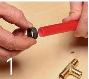
Slide a copper crimp ring onto the tubing, then insert the fitting into the tubing, making sure it's fully seated.
