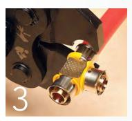
Align the PEX press tool squarely over the fitting sleeve.
