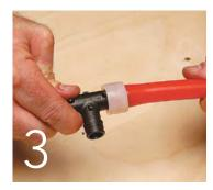
Remove the tool and insert the fitting so its shoulder is snug against the sleeve. The fitting should be secure within seconds.
