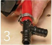
Align the clamp so it's about <sup>1</sup>/<sub>8</sub> in. to <sup>1</sup>/<sub>4</sub> in. from the end of the tubing. As with crimping, the clamp should be aligned over the fitting's central ribs.
