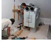
Taming the tubes. One of the carpenters cuts the Zehnder duct tubes to length before connecting them to the manifold.
