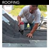
**Dried in.** Zip System sheathing and tape dries the roof in early. A synthetic underlayment adds an additional layer of protection before shingling.
