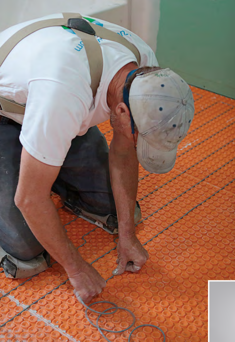
Beneath the surface. Electric radiant cables gently warm the tile so the soft, smooth soapstone is comfortable underfoot year-round.
