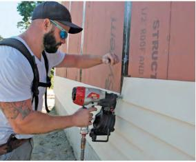
Barely visible fasteners. All trim boards are attached with FastenMaster's Cortex system of screws and Boral plugs. The siding is blindnailed with a single visible face nail at the bottom edge at each butt joint.
