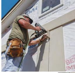
Use spacers for consistency. Once you've determined your layout, use spacers to maintain a consistent gap between boards and keep your layout on track. Here we used ½-in.-thick scraps of plywood.
