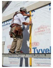
Work from the middle out. To start, measure the wall and find its center. Then draw a plumb line from top to bottom through the centerpoint as a reference for the first board.
