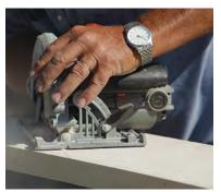
Same old tools. Poly-ash trim can be cut with standard carpentry tools using carbide-tipped blades. Dedicate blades to this material, though, because after cutting poly ash, a blade isn't much good for cutting wood.
