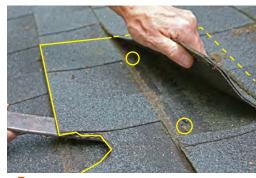
**Pry it out.** Using the flat bar, pry the bad shingle up from below. The idea is to force the shingle to tear around the nails holding it down.
