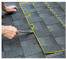
Pry with care. Loosen the shingle to be replaced by sliding a flat bar between it and the shingle below, working from one side to the other. Try to avoid damaging the shingle below by cutting the asphalt tabs with the bar end rather than just prying upward.
