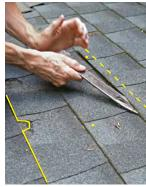
Repeat the process. Next, use the pry bar to loosen the two rows of shingles above the one to be replaced. Again, focus on not damaging these shingles. To provide access for nailing, you'll need to loosen these rows at least half a shingle width to each side of the one you're replacing so they can be lifted up without breaking.
