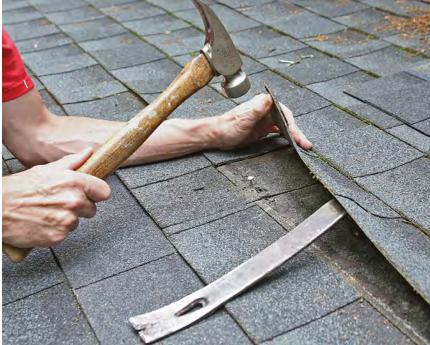
Prive it home. Nail the new shingle to the roof and re-nail the upper shingle, staying an inch or so away from the existing nail holes. Follow the shingle manufacturer's instructions regarding where to nail.
