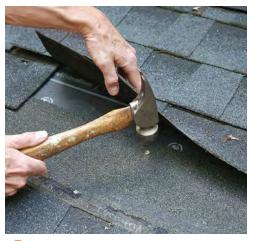
Flush the existing nails. With the bad shingle out, drive the protruding nails down flush with the shingle below. They can also be pulled, but that causes more damage to the shingle below.
