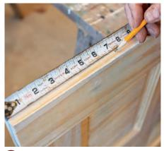
Locate the hinges. Mark the hinge locations on the door and on the jamb, locating the hinges about <sup>3</sup>/<sub>32</sub> in. lower on the jamb to create a clearance space between the door and the head jamb when the door is hung.
