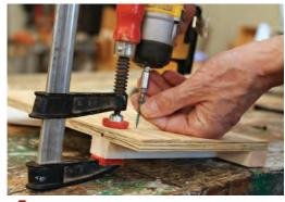
Attach the side fences. Clamp the side fences to the plywood along the lines made in step 2, and screw them home from the back.
