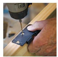
12 Attach the hinges. The hinges should fit in the mortises with very little slop, and be flush with, or ever so slightly proud of, the edge of the door and the face of the jamb.
